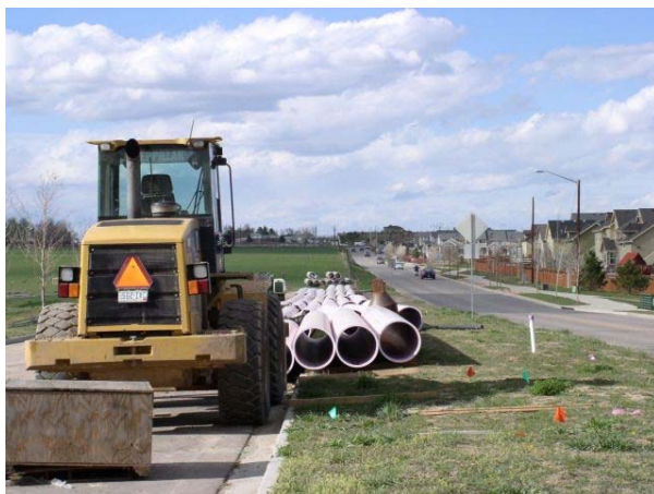
Staging for reuse water line installation.
