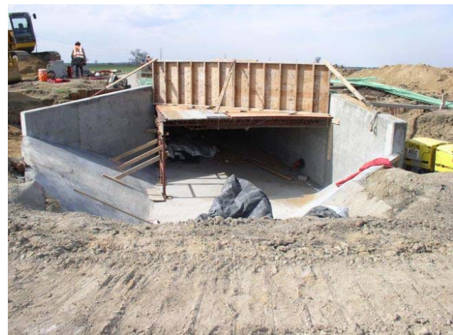
Weld County Road 6 bridge construction.
